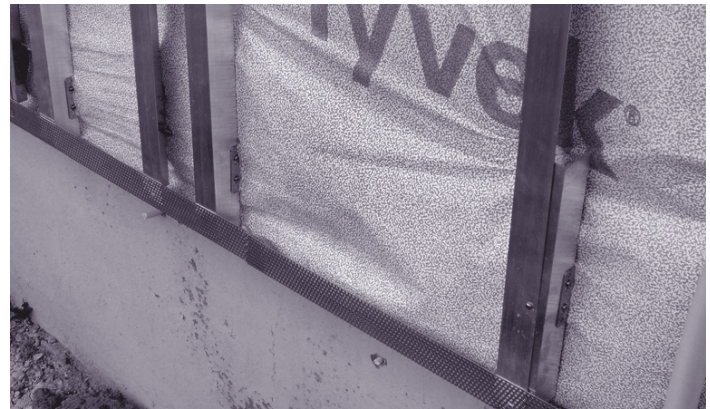
Dilatation – grid of aluminium or zinc-coated profiles
